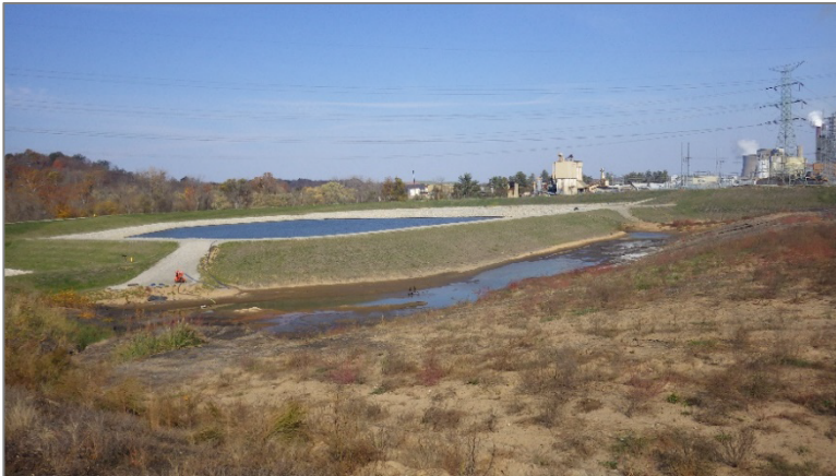
Photo 14, Point 14 Boiler Slag Pond – Southwest Divider Dike – Divider dike elevation looking at LVWTS basins.
