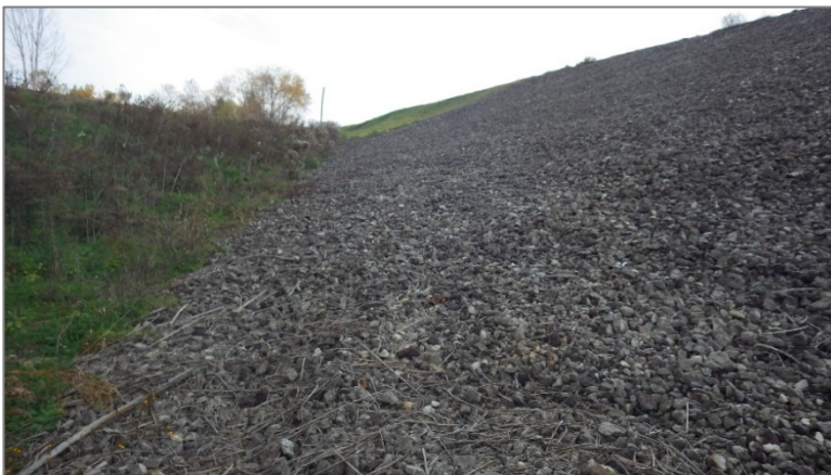
Photo 27, Point 26 Northwest Exterior Slope – Edge of riprap protection
