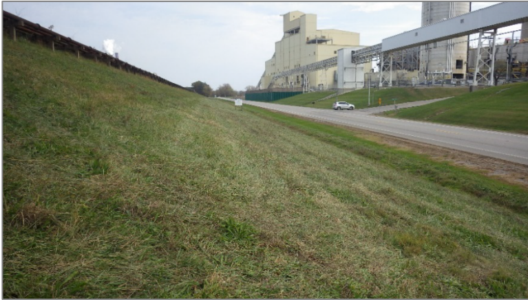
Photo 37, Point 36 Southeast Exterior Slope – Looking northeast.
