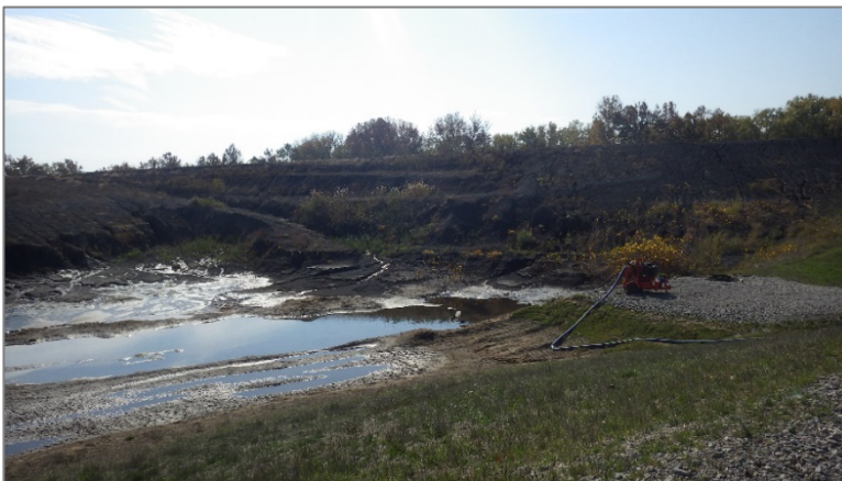
Photo 12, Point 12 LVWTS Secondary Basin – Interior dike elevation.
