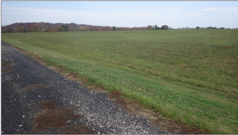
Photo 43, Point 42 Southeast Exterior Slope – Slope tie-in on northeast side.
