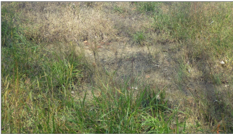
Photo 8, Point 8 Boiler Slag Pond – Southeast Exterior Slope – Bare spot near the toe.
