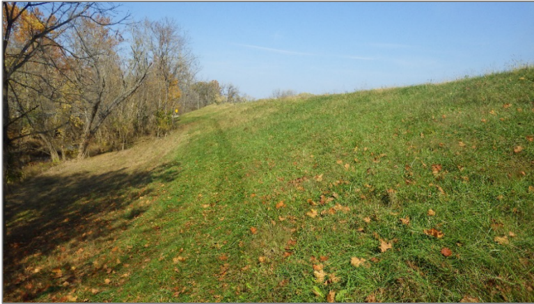
Photo 19, Point 18 LVWTS – West Exterior Slope – Looking north.
