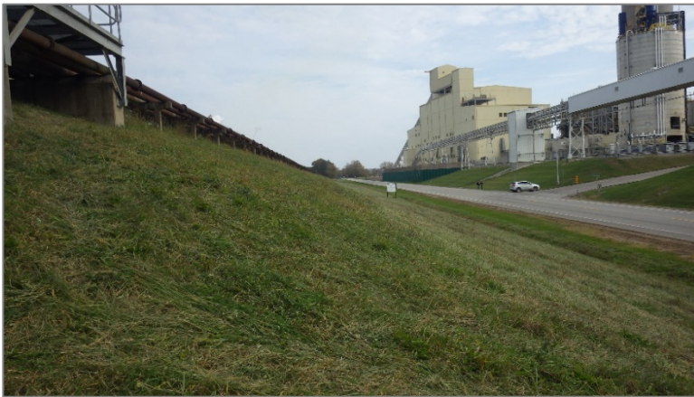
Photo 35, Point 34 Southeast Exterior Slope – Looking northwest.
