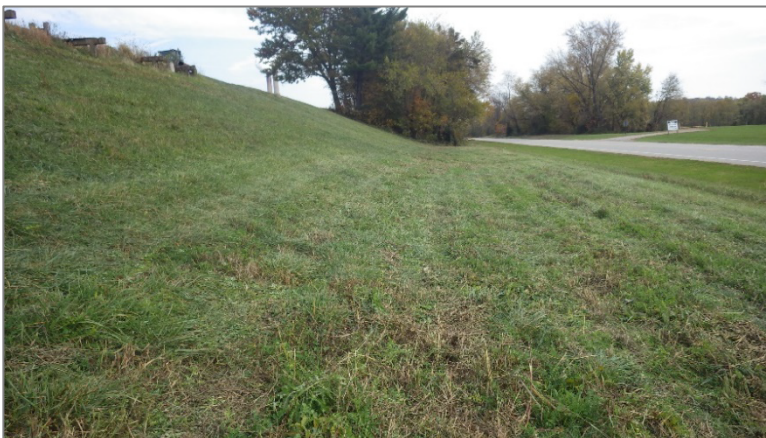
Photo 42, Point 41 Southeast Exterior Slope – Slope tie-in location.
