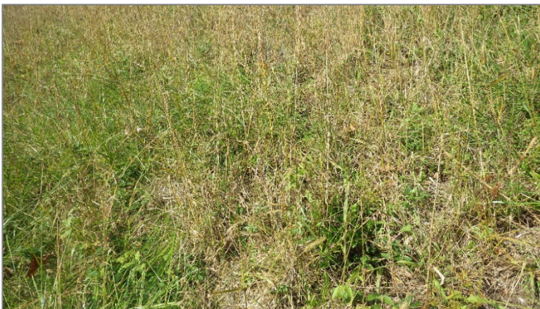
Photo 9, Point 9 Boiler Slag Pond – Southeast Exterior Slope – Animal burrow near the toe.
