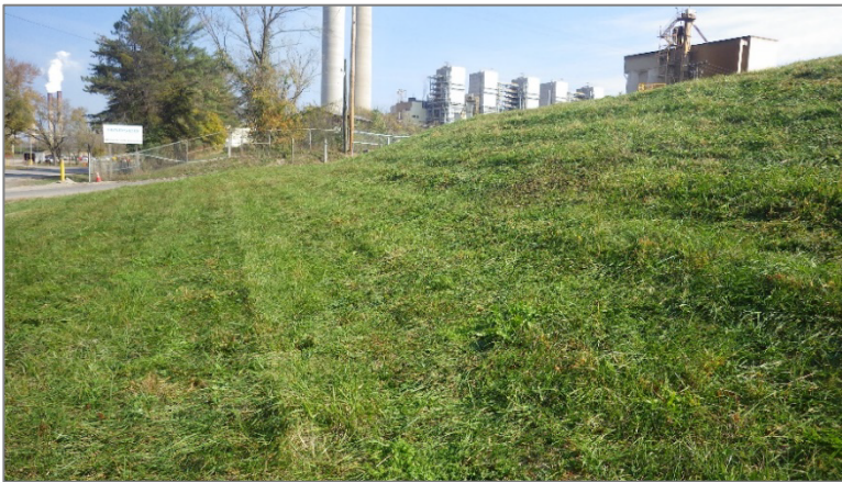
Photo 23, Point 22 LVWTS – West Exterior Slope – Looking north at Primary Basin.
